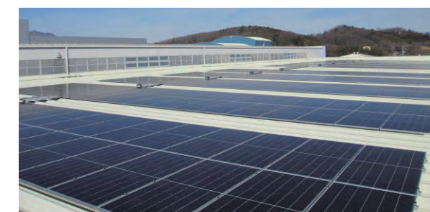
Solar panels additionally installed in Tomioka Plant
