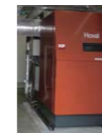
LPG boiler for air conditioning installed in fiscal 2014
